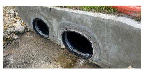
**LOW HEAD LOSS IN-LINE RUBBER CHECK VALVES**
