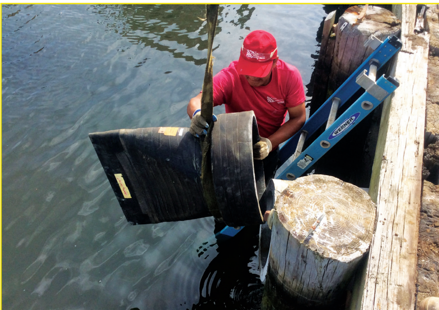
A 24" ProFlex 730 slip on valve being readied for install
