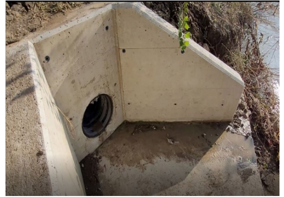
Final installation of valve in headwall
