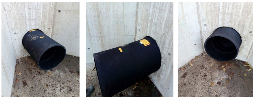
Progress photos of the Style 790 installation
